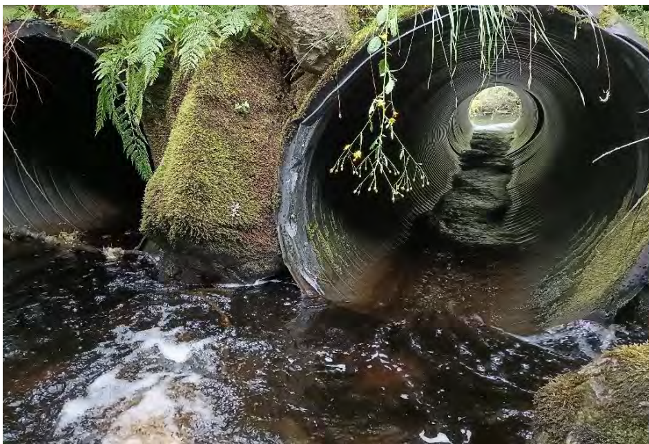
Plate 7-3 View downstream though Forestry Culvert, downstream of Flaggy Bridge (30 August 2024)
